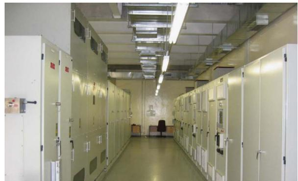
Fig. 2. (Left) ASD. (Right) Excitation and control panels.
