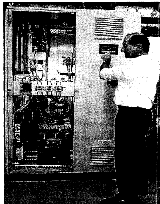
Fig. 9: 1 MVA AVC unit
