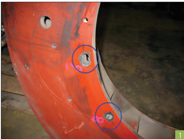
One damaged fan bolt hole and another with no damage.
